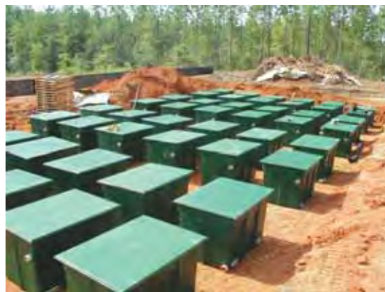
Figure 6-5: Construction of the 20,000 GPD Decentralized Wastewater Treatment System at Snow Road, Showing Installation of Textile Filter Units
