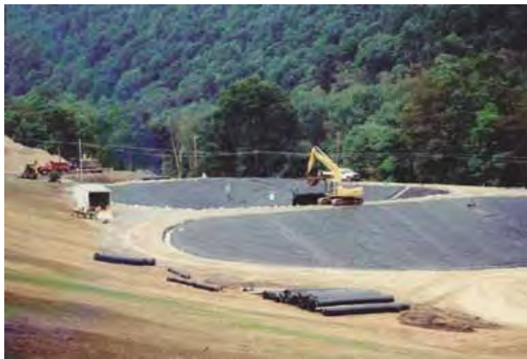
Figure 12-4: Construction of the Aerated Lagoon Treatment System for Riddlesburg and the Six Mile Run Valley
