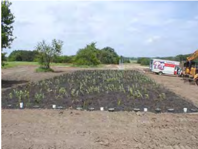
Figure 11-3: The West Wetland Cell of the EWTS at The Fields of St. Croix, Phase II
