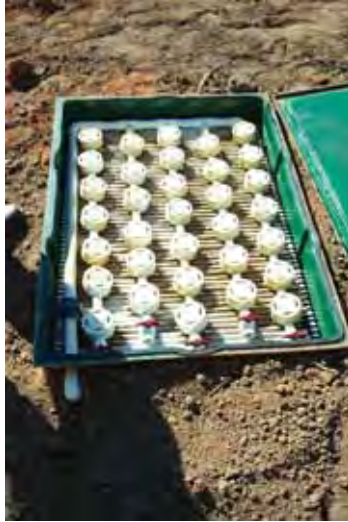
Figure 6-6: Close-Up View of the Filter Media and Effluent Distribution Systems
