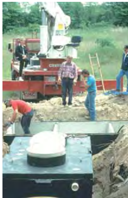
Figure 13-4: Construction of a Demonstration Denitrifying Sand Filter System for the Grocery Store on Washington Island
