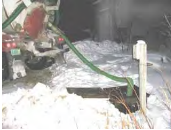
Figure 13-3: Pumping a Holding Tank on Washington Island
